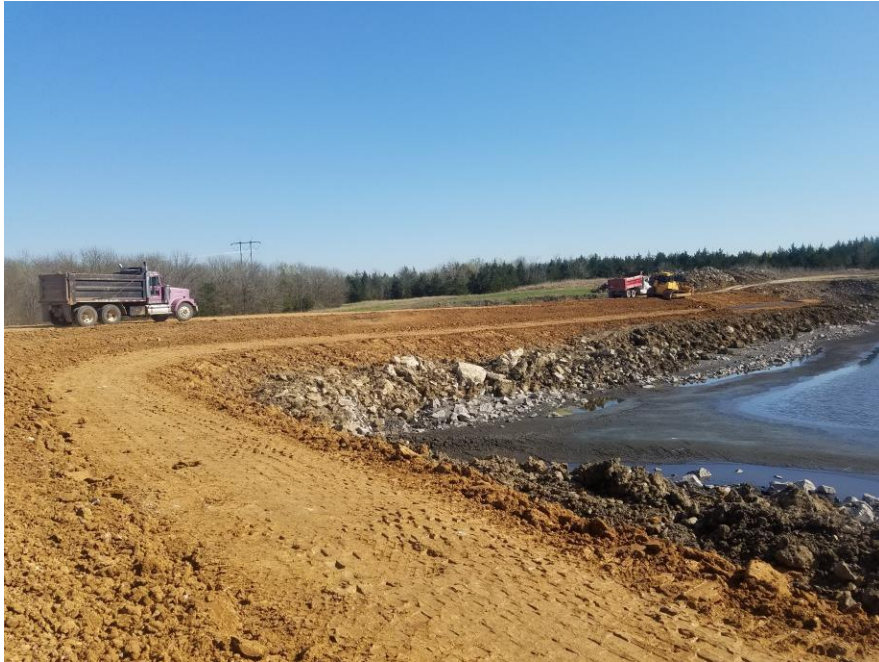
FIGURE 9: ADDITIONAL FILL IS DELIVERED AND PLACED ON THE EMBANKMENT
