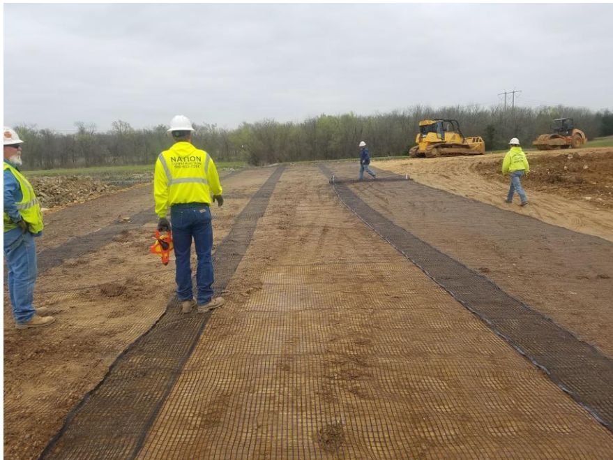
FIGURE 10: FIRST LAYER OF GEOGRID FOR THE UPPER 8 FEET OF THE EMBANKMENT
