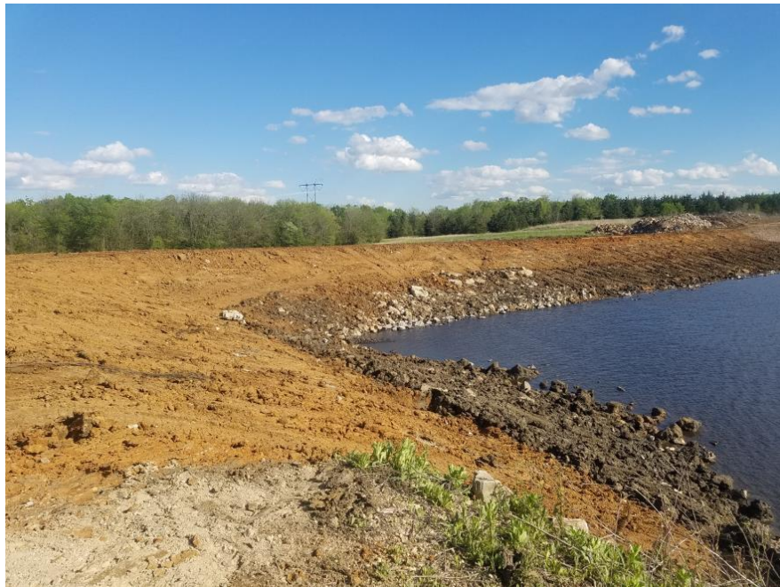
FIGURE 13: FINAL LAYER OF FILL WAS PLACED ON APRIL 5, 2017
