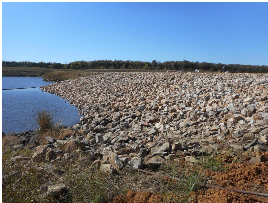
FIGURE 23: COMPLETION OF CCR UNIT 2 EASTERN EMBANKMENT WITH RIPRA PROTECTION
