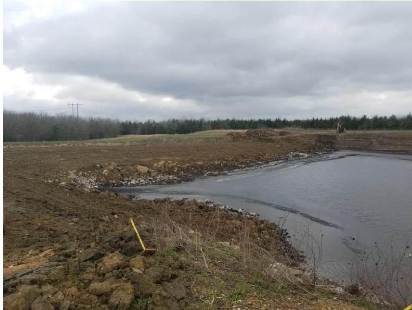
FIGURE 4: REMOVAL AND STOCKPILING OF THE EXISTING RIPRAP
