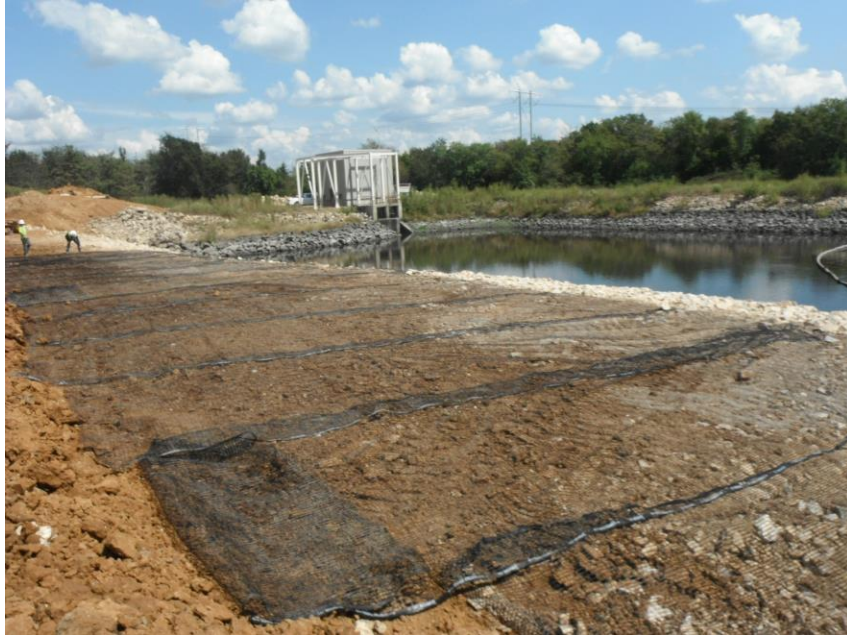
FIGURE 19: PLACEMENT OF GEOGRID TO SECURE ROCK TOE BERM TO EMBANKMENT
