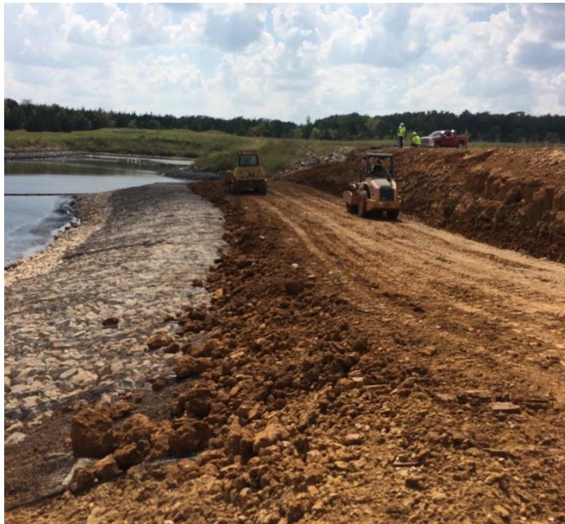
FIGURE 20: PLACEMENT OF ADDITIONAL FILL BENCHED INTO THE EMBANKMENT
