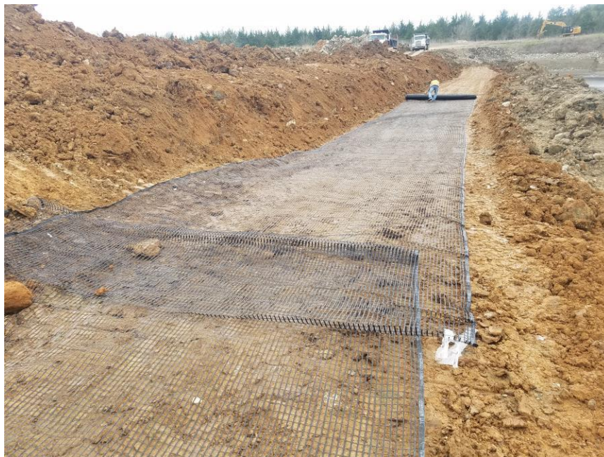
FIGURE 8: THE TRENCH BACKFILLED AND SECURED TO THE EMBANKMENT WITH GEOGRID
