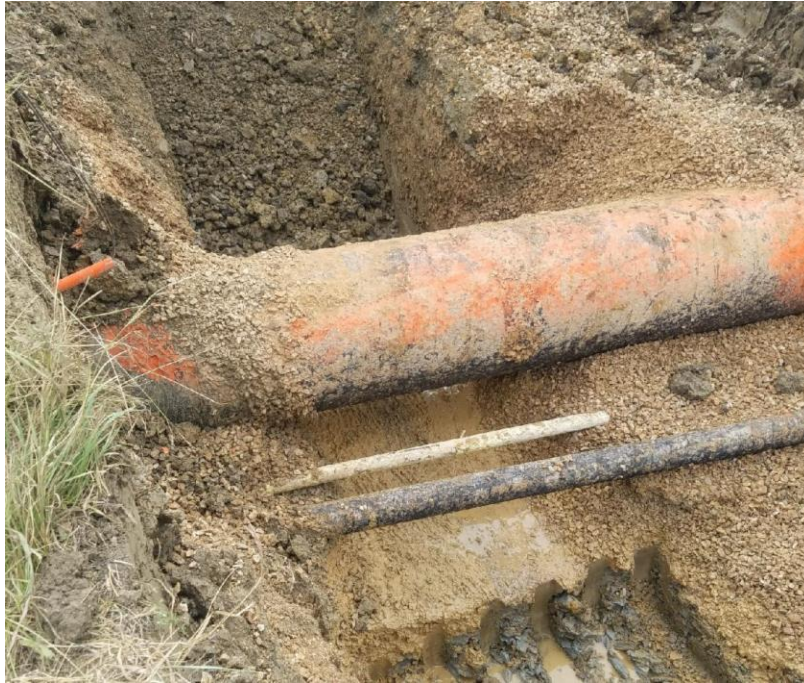
FIGURE 21: HYDROVAC EXCAVATION TO EXPOSE BURIED UTILITIES
