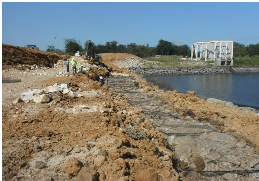
FIGURE 18: PLACEMENT OF ROCK AND GEOGRID IN ROCK TOE BERM
