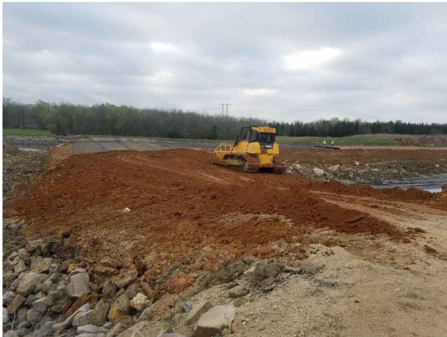
FIGURE 11: FILL PLACED OVER GEOGRID
