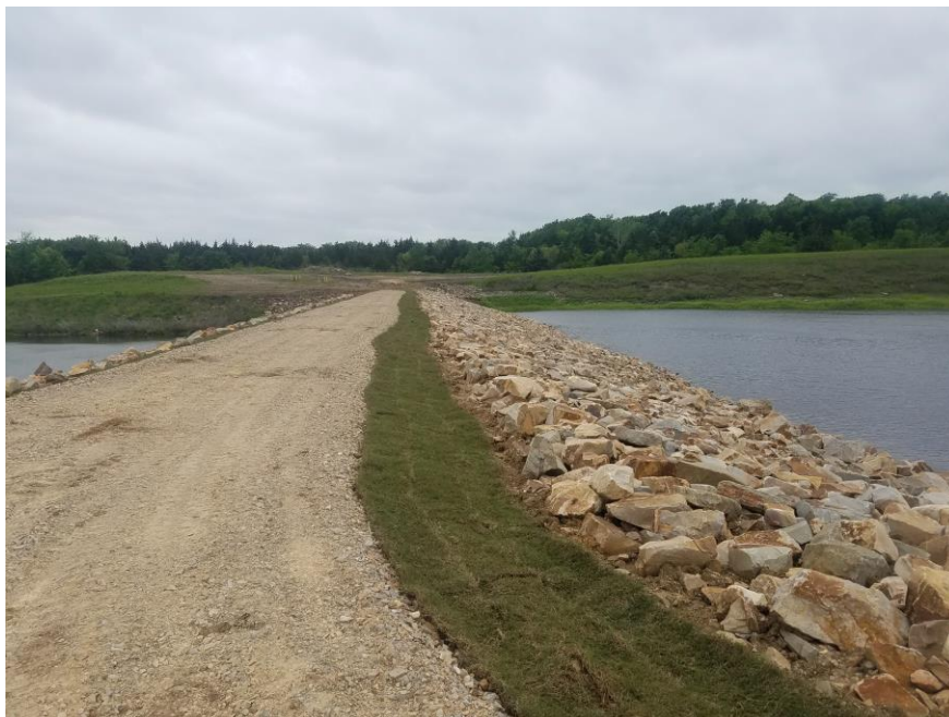
FIGURE 15: COMPLETED CCR UNIT 3 EASTERN EMBANKMENT FOR PHASE 1 OF THE PROJECT
