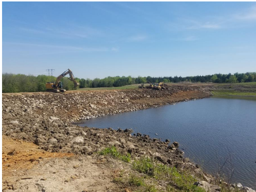
FIGURE 14: PLACEMENT OF RIPRAP FOR SLOPE PROTECTION
