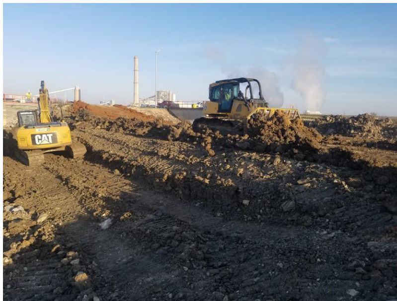
FIGURE 5: BEGINNING EARTHWORK OPERATIONS
