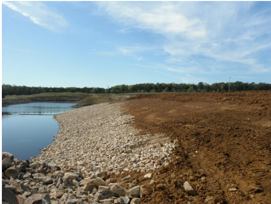
FIGURE 22: COMPLETION OF CCR UNIT 2 EASTERN EMBANKMENT PRIOR TO PLACEMENT OF RIPRAP
