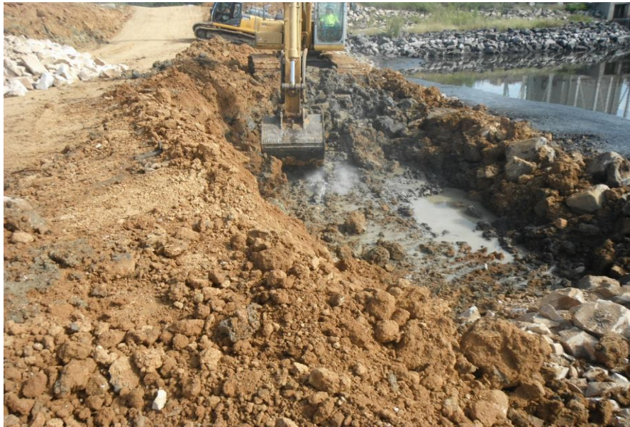
FIGURE 17: EXCAVATION OF TOE TRENCH FOR ROCK TOE BERM
