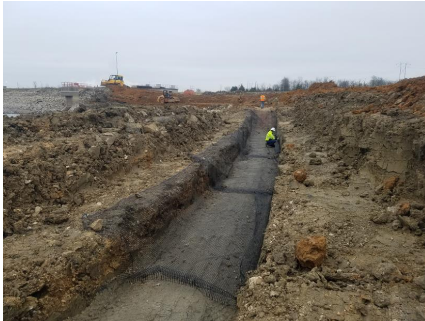
FIGURE 7: REINFORCING THE TRENCH WITH GEOGRID
