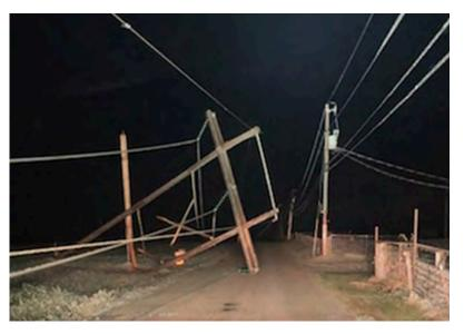
High voltage transmission structures and substations were no match for the heavy ice accumulations. Numerous transmission structures were twisted and mangled, with long stretches of downed or damaged structures in some areas.
