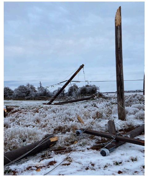
The heavy ice was no match for transmission structures and power lines that succumbed to the weight of the one to four inches of ice across parts of Oklahoma. Pictured above is damage along the Hydro to Eakly line, taken by Kenny Flood, a WFEC journeyman station technician.
